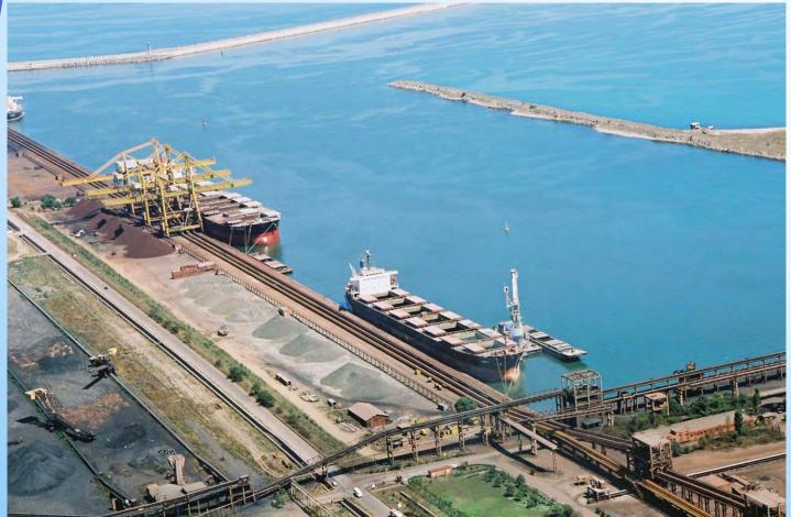
COMVEX is the only terminal for the operation of solid bulk raw materials in the Black Sea area that is able to cater Cape size vessels of up to 220.000 tdw, having an unloading line at the maritime quay formed of 5 berths with a total length of 1.400 m and water depth comprised between 10.8 and 18.5 m. Those materials are:
