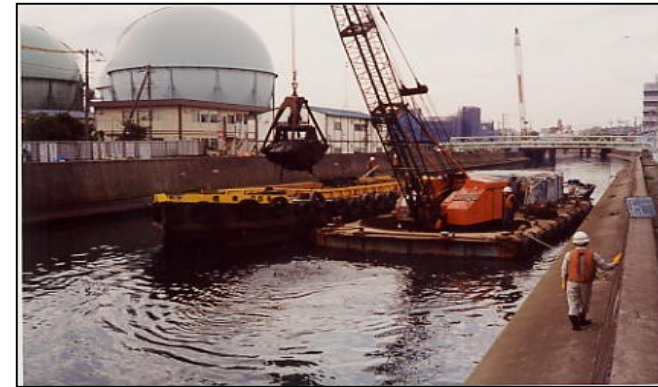
Dredging of Sludge
