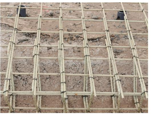
GFRP rebar for concrete at grade (flat work) by the coast-line
