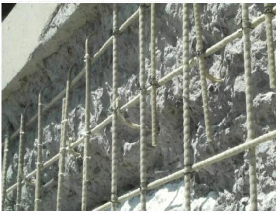
Grid of 19mm (#6) GFRP bars doweled and epoxied in place
