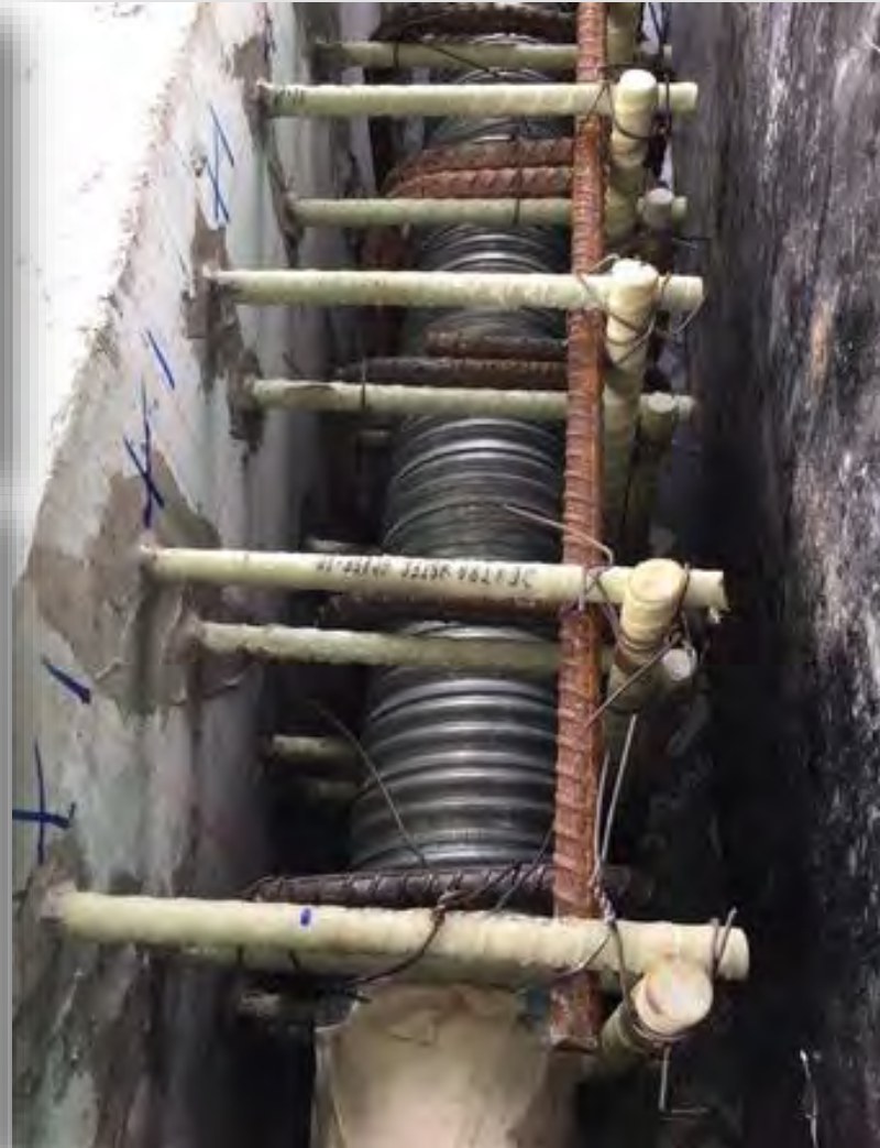
Concrete with GFRP dowels & post-tensioned steel bar
