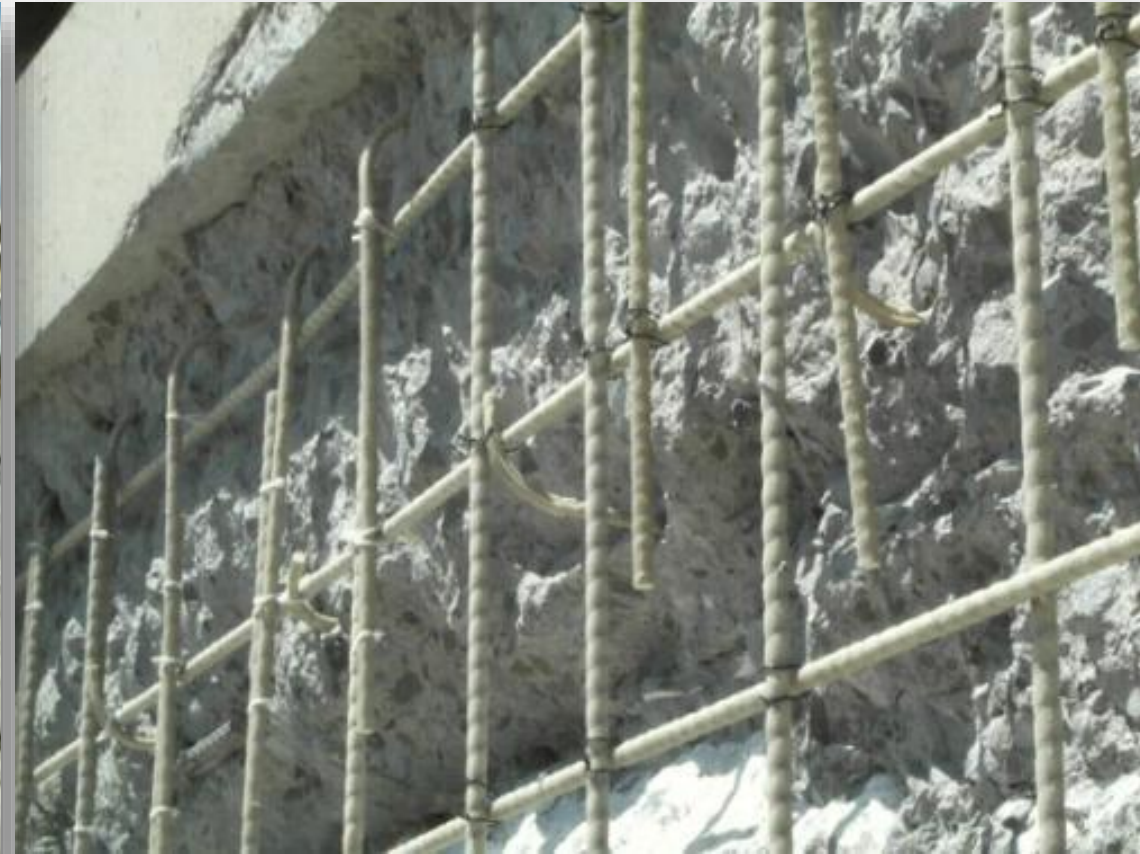
Grid of 19mm (#6) GFRP bars doweled and epoxied in place
