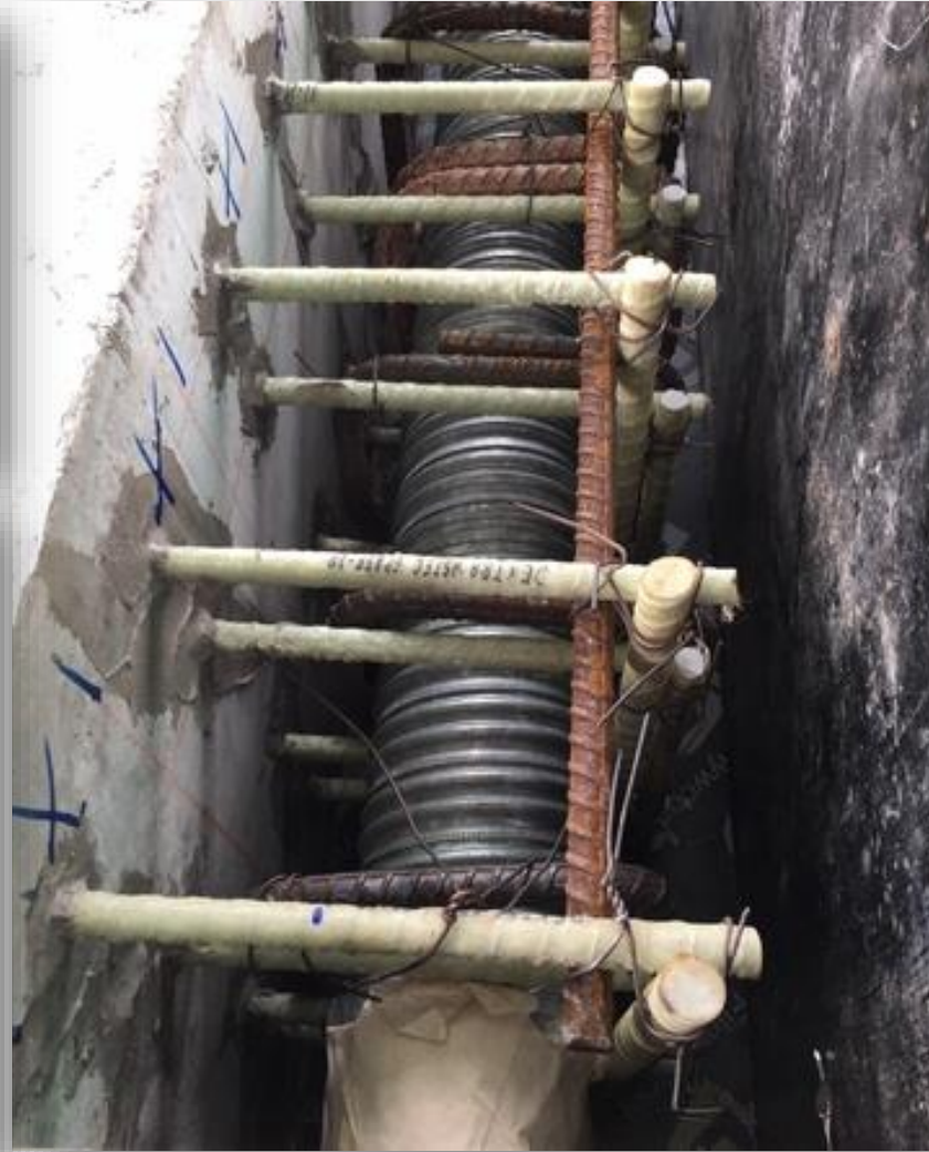
Concrete with GFRP dowels & post-tensioned steel bar
