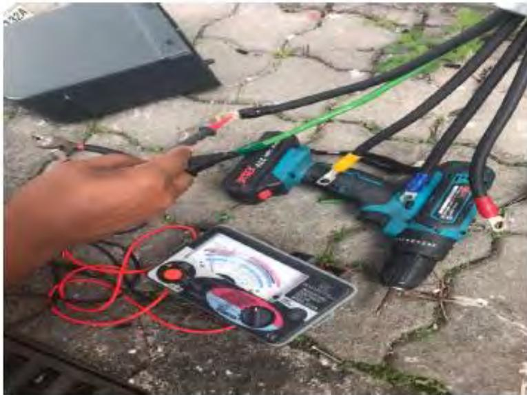
Installation of Weather Station, Megger Test, Insulation Test and Continuity Test at Warehouse FZ5
