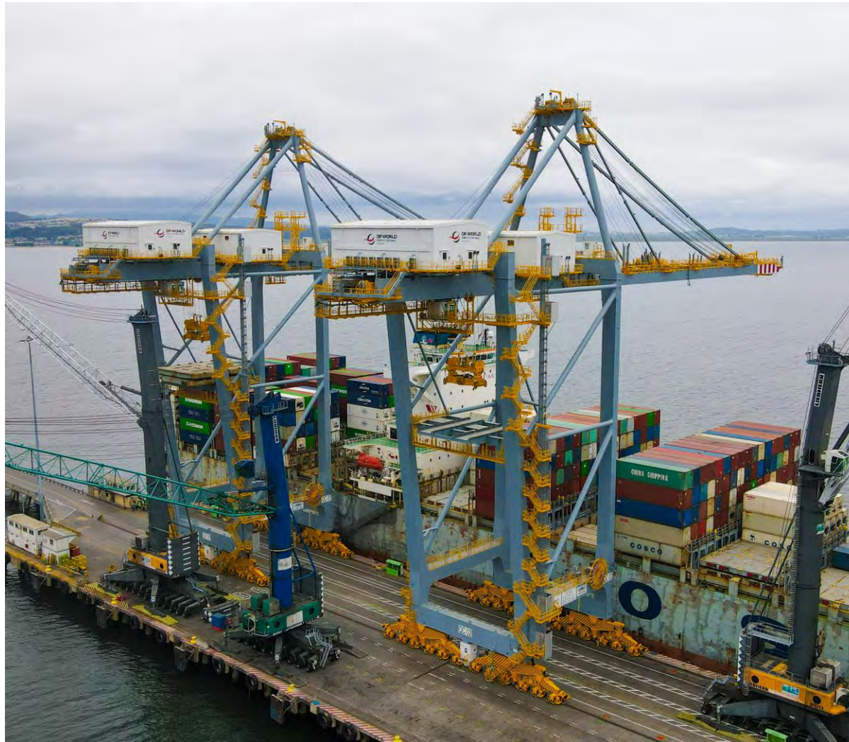
DP World, two Super Post Panamax ship-to-shore (STS) cranes at its Lirquén Chile terminal.
