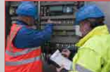
Inspection and maintenance
