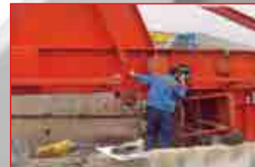
Refurbishment and upgrades
