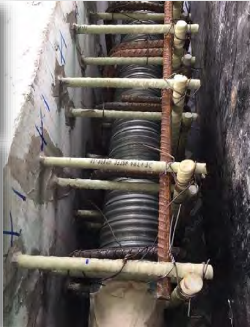
Concrete with GFRP dowels & post-tensioned steel bar
