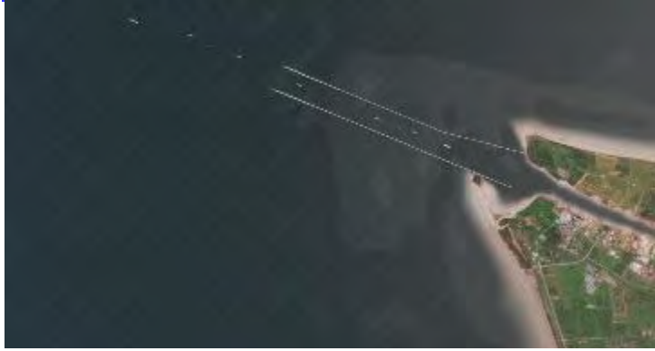
Phase 1 : Kuala Baram Access Channel (2024-2027)
