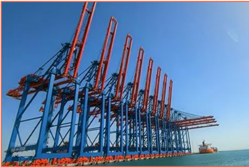
2025 marked the inauguration of SCCT's 2.2 million TEU expansion.
