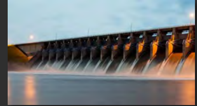
Renewable Energy & Power Generation
