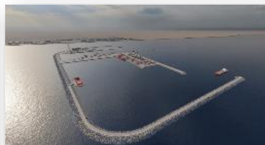
PORT OF DAKHLA ATLANTIQUE
