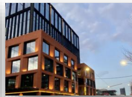
CAMCO Australia Office
