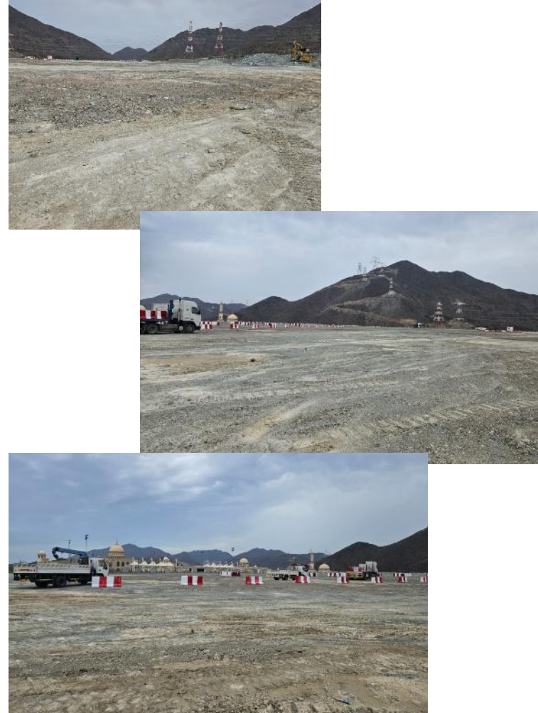
Construction: 3 rd -4 th Week into the crisis
