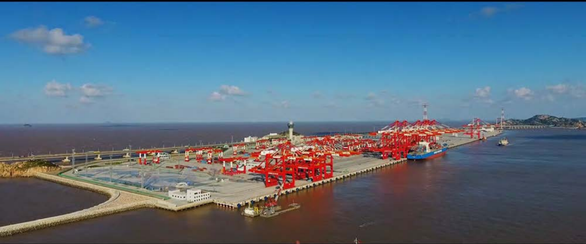
上海洋山四期自动化码头 Shanghai Yangshan Phase IV automated terminal
