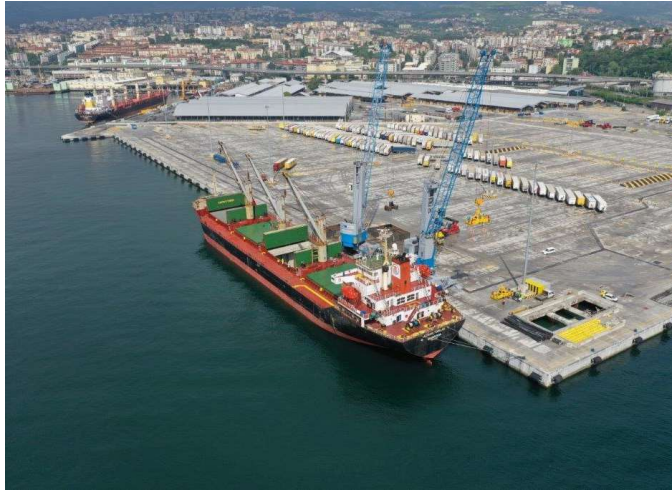
Pig iron unloading for neighboring steel mill
