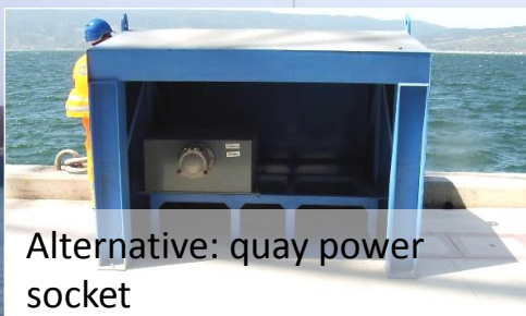
Underground quay switch cabinet
