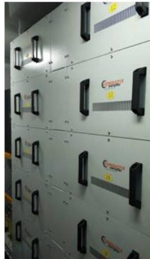
Battery modules inside the housing
